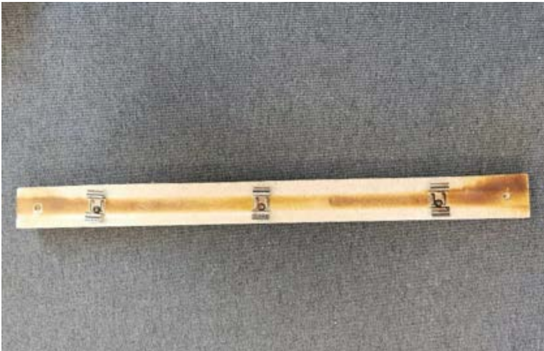
Photo No. 2 Damages on the wooden lath
